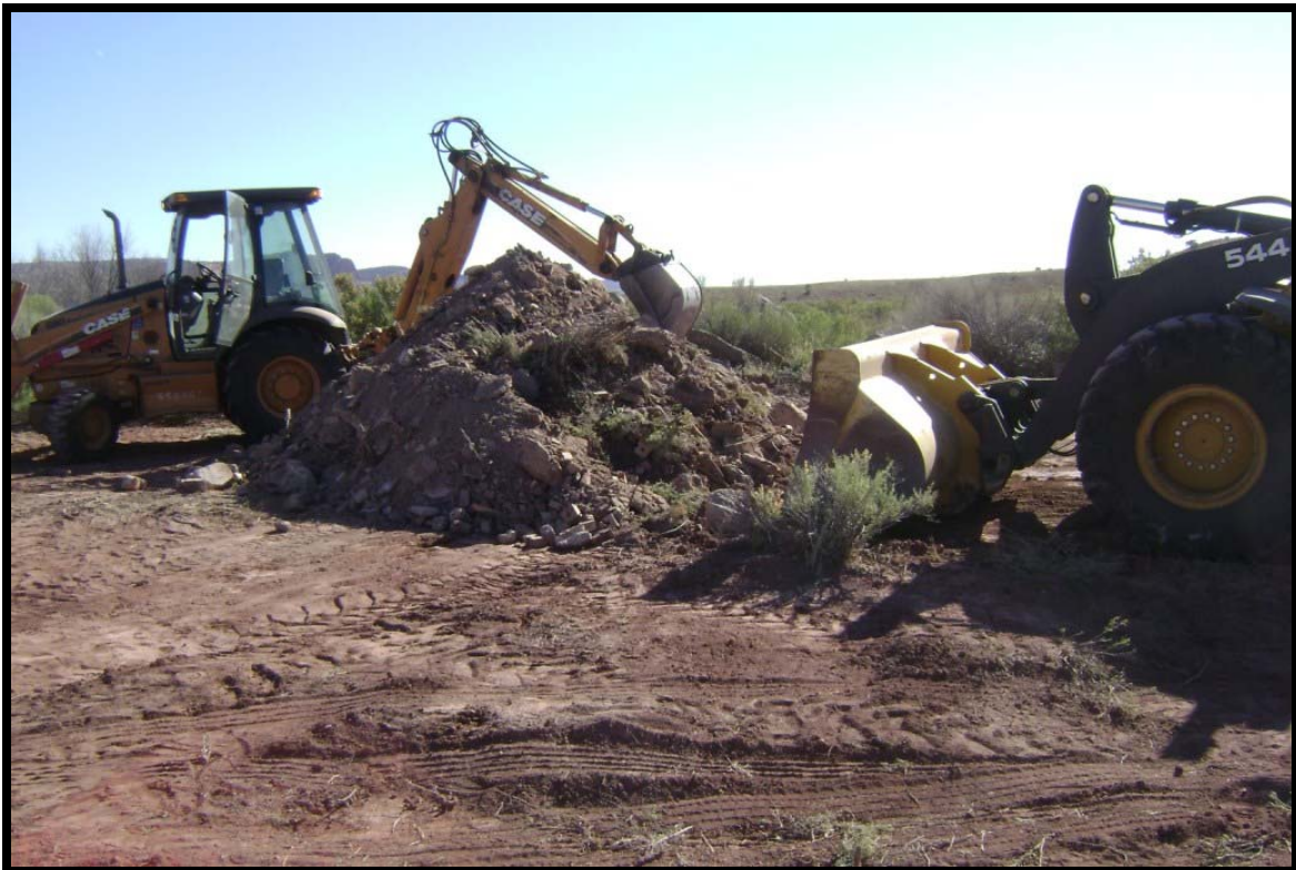
Parcel 12 / AOC 93 – Bivouac and Tank Training Area – South debris pile area removal
