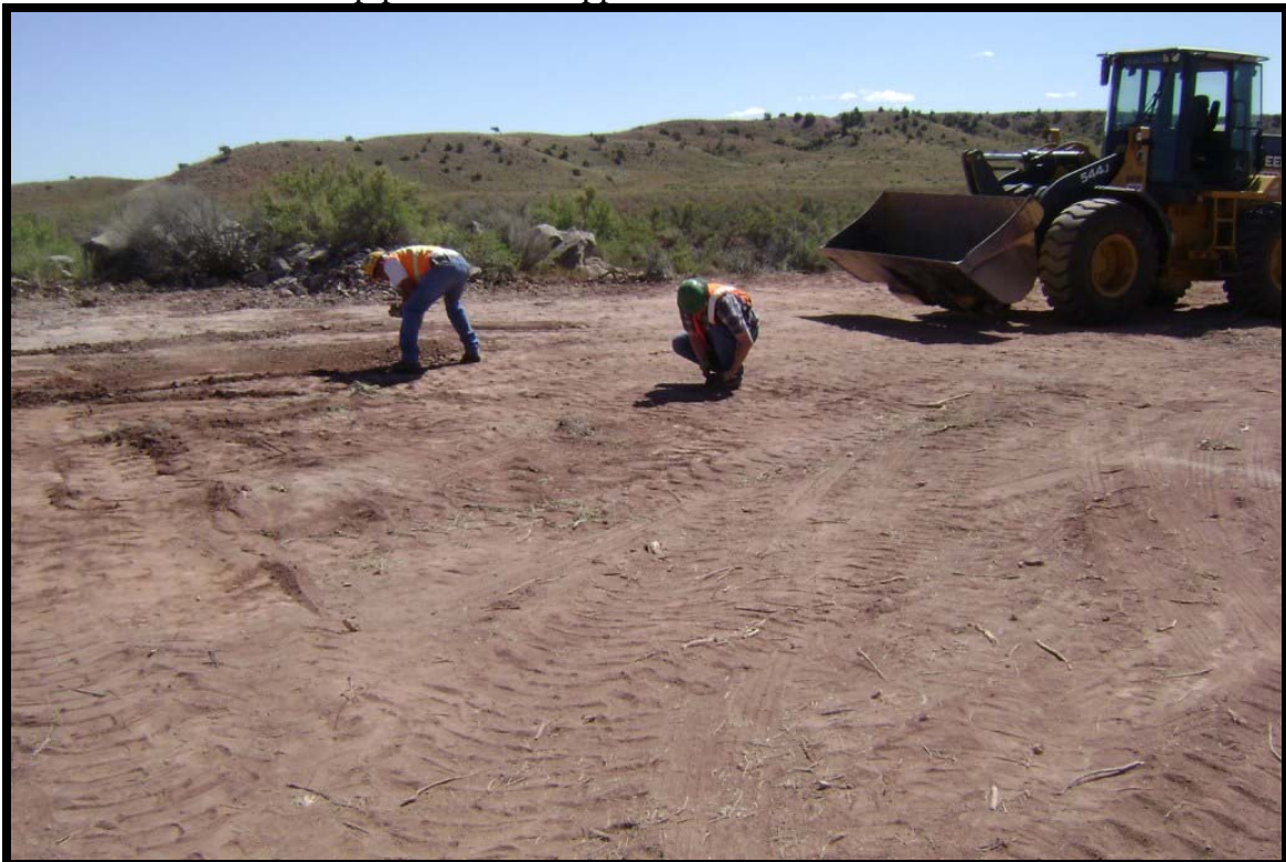
Parcel 12 / AOC 93 – Bivouac and Tank Training Area – South debris pile area removal - final sweep for remaining debris
