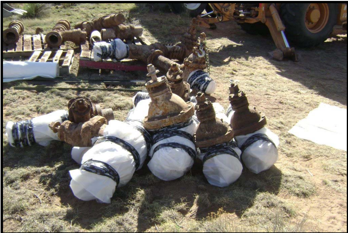
Parcel 12 / AOC 93 – Bivouac and Tank Training Area – North debris pile area removal - asbestos contaminated pipe double wrapped and sealed
